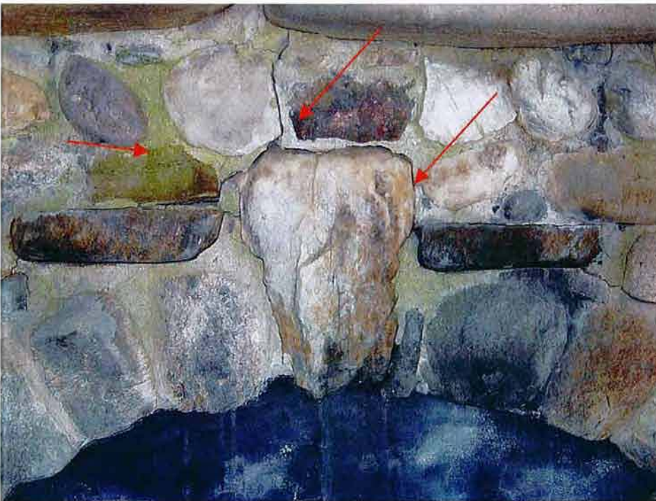
Photos 19 & 20: Damage to fireplace. The bio-growth that is evidence of water intrusion can be cleaned from the surfaces of the exposed chimney column. The cracks that have appeared between the large pebbles, in the brick of the firebox and in the cast concrete hearth can be filled, with care being taken to match the color and texture of the existing mortar.
