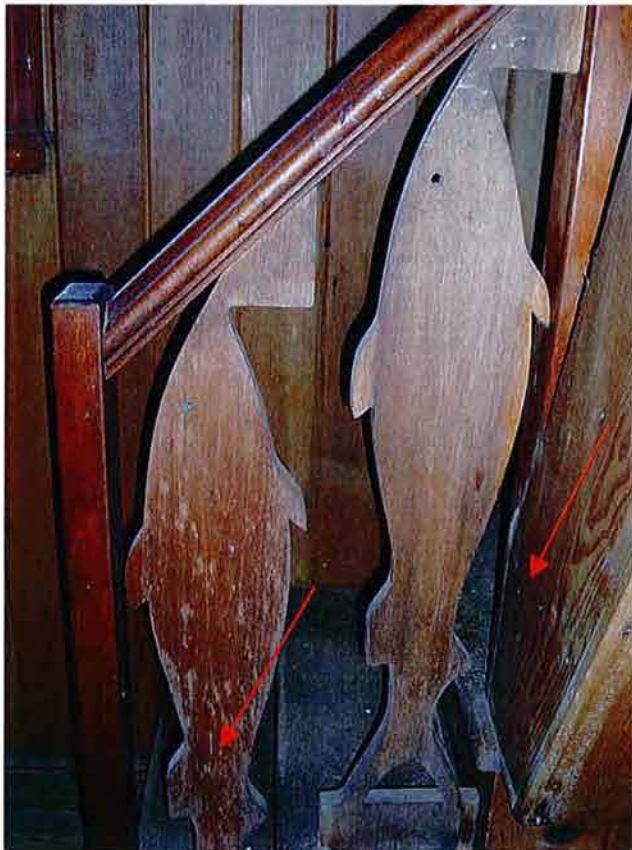
Photos 23 & 24: Interior finishes. Many interior finishes are soiled and unprotected. All wood surfaces will be cleaned and refinished with a clear protective coating. All historical applications will be restored where appropriate.
