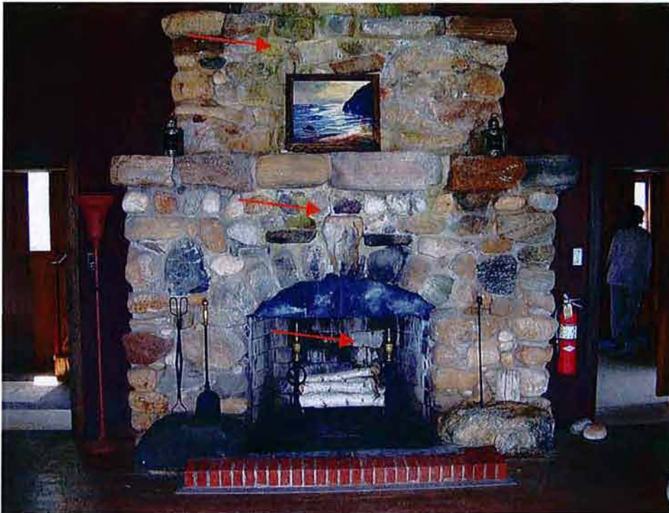
Photos 19 & 20: Damage to fireplace. The bio-growth that is evidence of water intrusion can be cleaned from the surfaces of the exposed chimney column. The cracks that have appeared between the large pebbles, in the brick of the firebox and in the cast concrete hearth can be filled, with care being taken to match the color and texture of the existing mortar.
