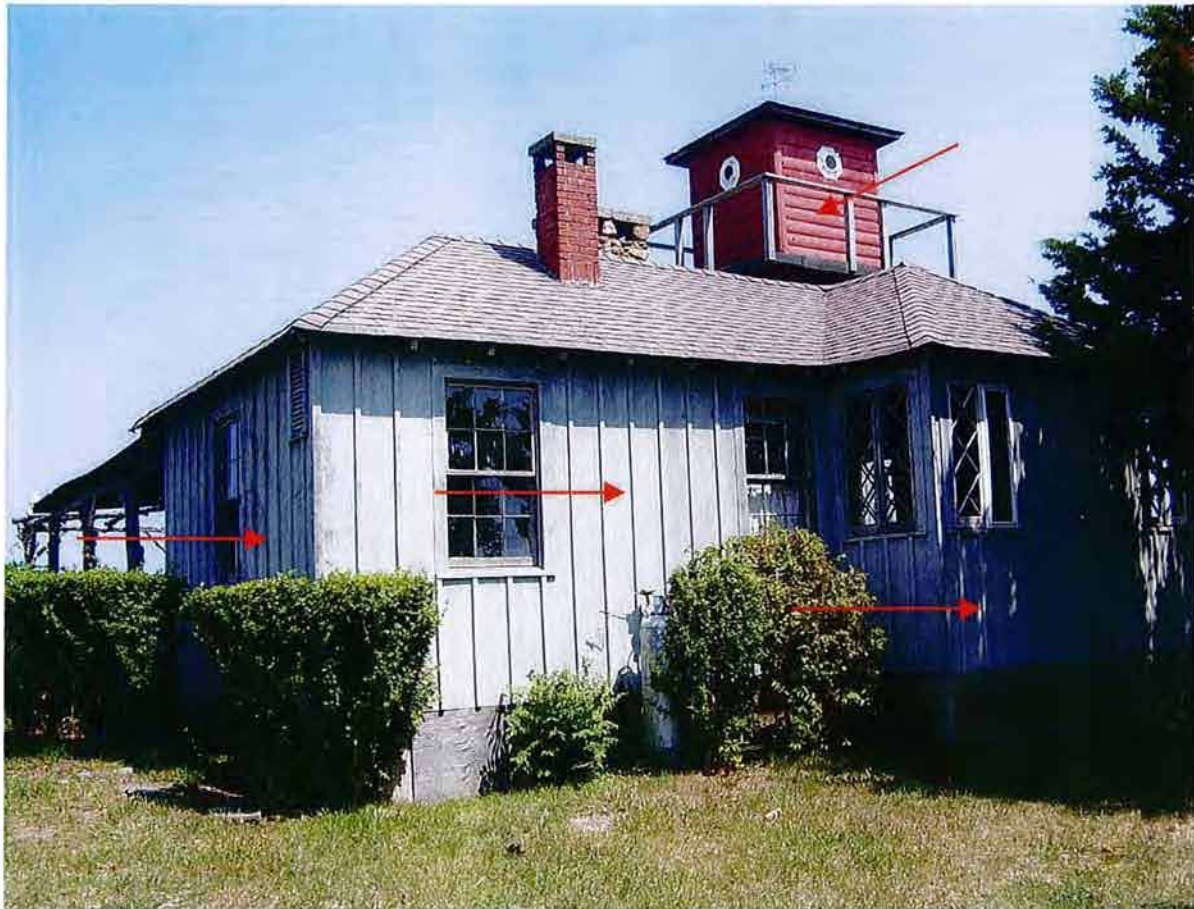
Photo 8: Non-historic board-and-batten siding is present throughout the exterior. These sections of the building in which original siding has been removed will be restored; these include the bedroom and kitchen wings, as well as the tower. The specification for this siding is readily available (pieces have been saved and stored in the basement). New siding will be milled to match the original and installed using historic photographs as a guide.
