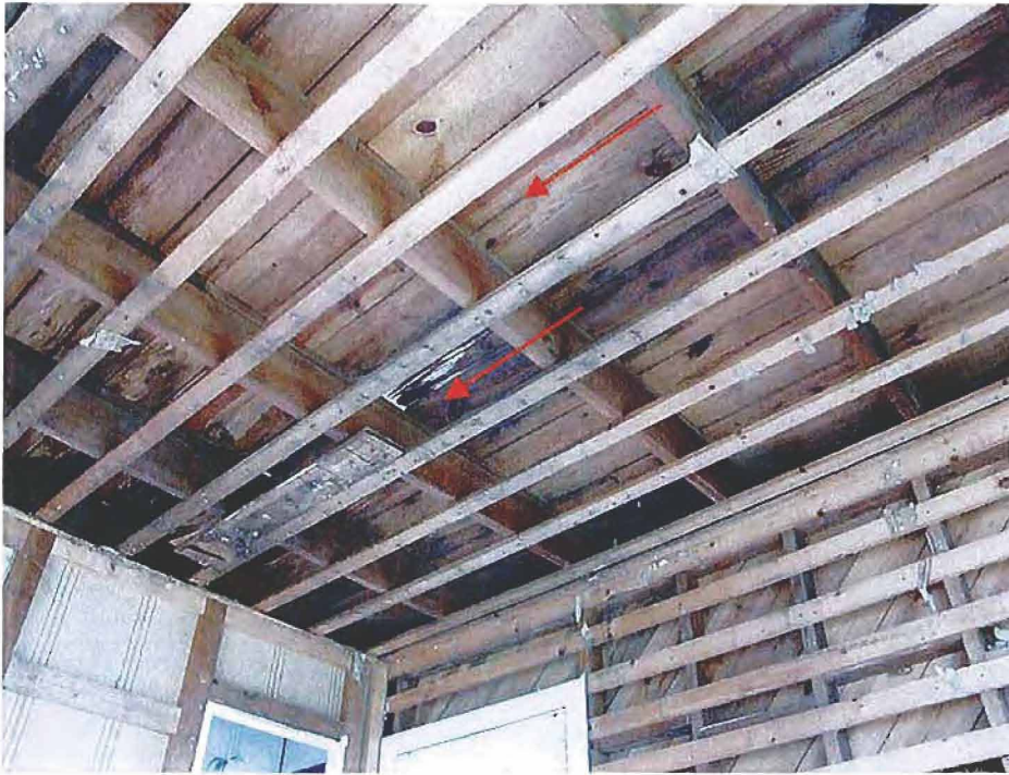
Photos 17 & 18: Walls & ceiling water damage. Water penetration has occurred in the east bedroom, resulting in failure of the ceiling and corner joints. Wall and ceiling coverings have been removed, and the areas will be cleaned and refurbished with historically appropriate material. Minor water damage has occurred in other areas of the Cabin, which will be repaired.
