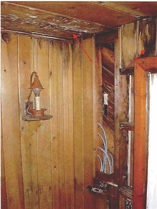
Photos 17 & 18: Walls & ceiling water damage. Water penetration has occurred in the east bedroom, resulting in failure of the ceiling and corner joints. Wall and ceiling coverings have been removed, and the areas will be cleaned and refurbished with historically appropriate material. Minor water damage has occurred in other areas of the Cabin, which will be repaired.
