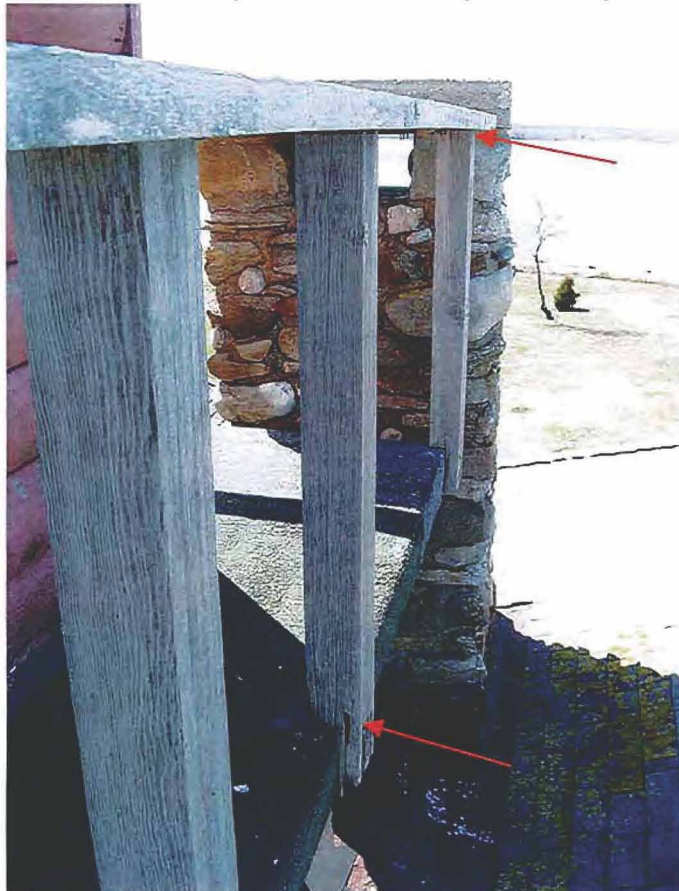
Photos 4 & 5: Tower balcony. The tower's narrow balcony is currently covered in an asphalt material that is deteriorating and cannot withstand foot traffic. The wooden railings are also unsafe. The balcony structure, decking and railing will be repaired to a safe condition.
