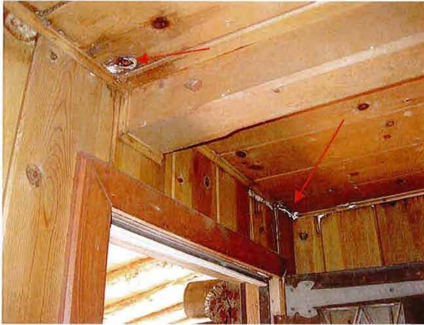
Photos 23 & 24: Interior finishes. Many interior finishes are soiled and unprotected. All wood surfaces will be cleaned and refinished with a clear protective coating. All historical applications will be restored where appropriate.
